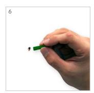
Insert wall plugs into the drilled holes, using a mallet if necessary.
